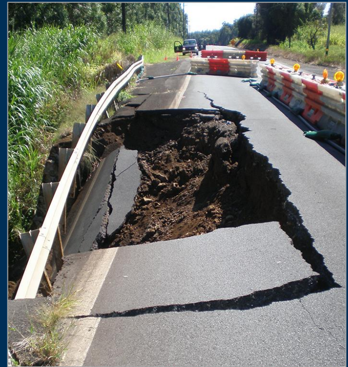
Highway 19, southeast of Kawāili Bridge.
