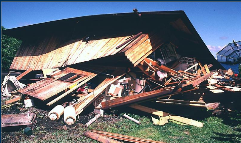
Collapsed home in Kalapana, Hawai'i. USGS photo.
